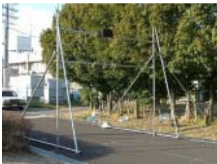
図5 スピーカ設置のためのやぐら Fig.5 Scaffold for speakers
