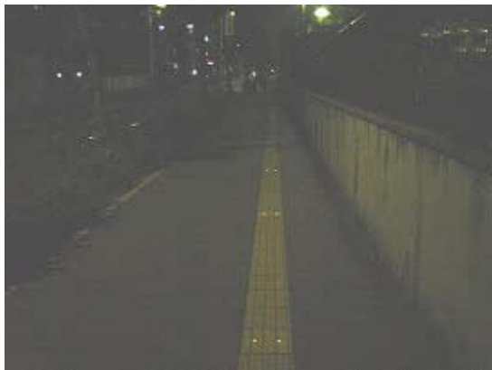
図1 事例1 - LED 内蔵誘導用ブロック Fig.1 Case1-Studded paving block with LED buried
