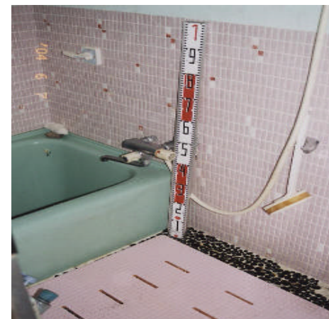
図11 改造前浴室 Fig.11 Bathroom before remodeling
