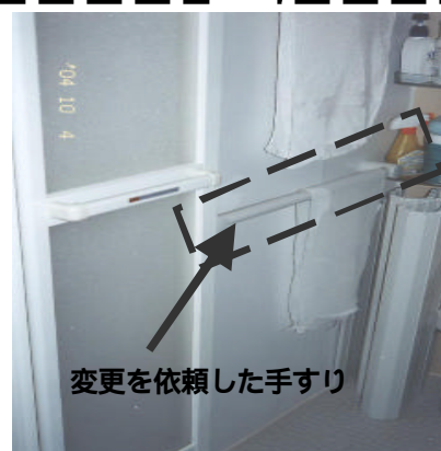
図14 改造後浴室 Fig.14 Bathroom after remodeling
