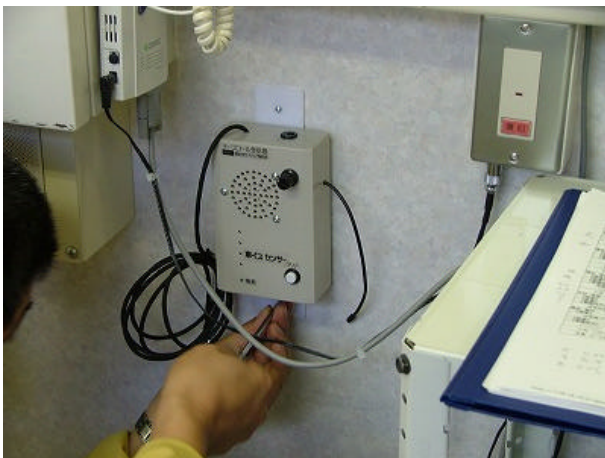
図12 無線式ナースコール受信機 Fig.12 Wireless receiver for nurse-call responding to some kind of specific alarms
