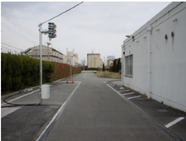
図12 屋外実験施設 Fig.12 The outdoor experiment system
