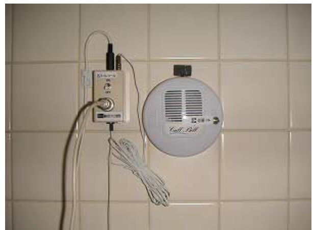
図12 作動スイッチと警報ブザー Fig.12 Operation switch and a buzzer
