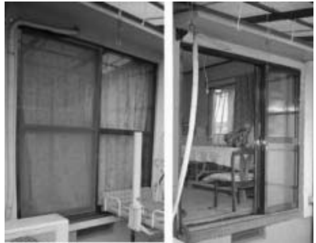
図4 掃出し窓(左:改造前,右:改造後) Fig.4 Remodel a window (Left: before, Right: after)
