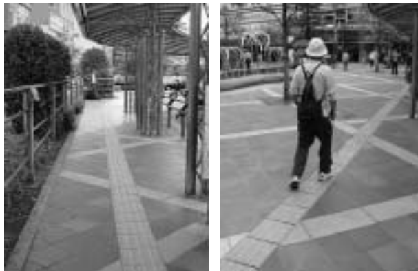
図12 駅前広場・1 Fig.12 In front of station Plaza (part1)
